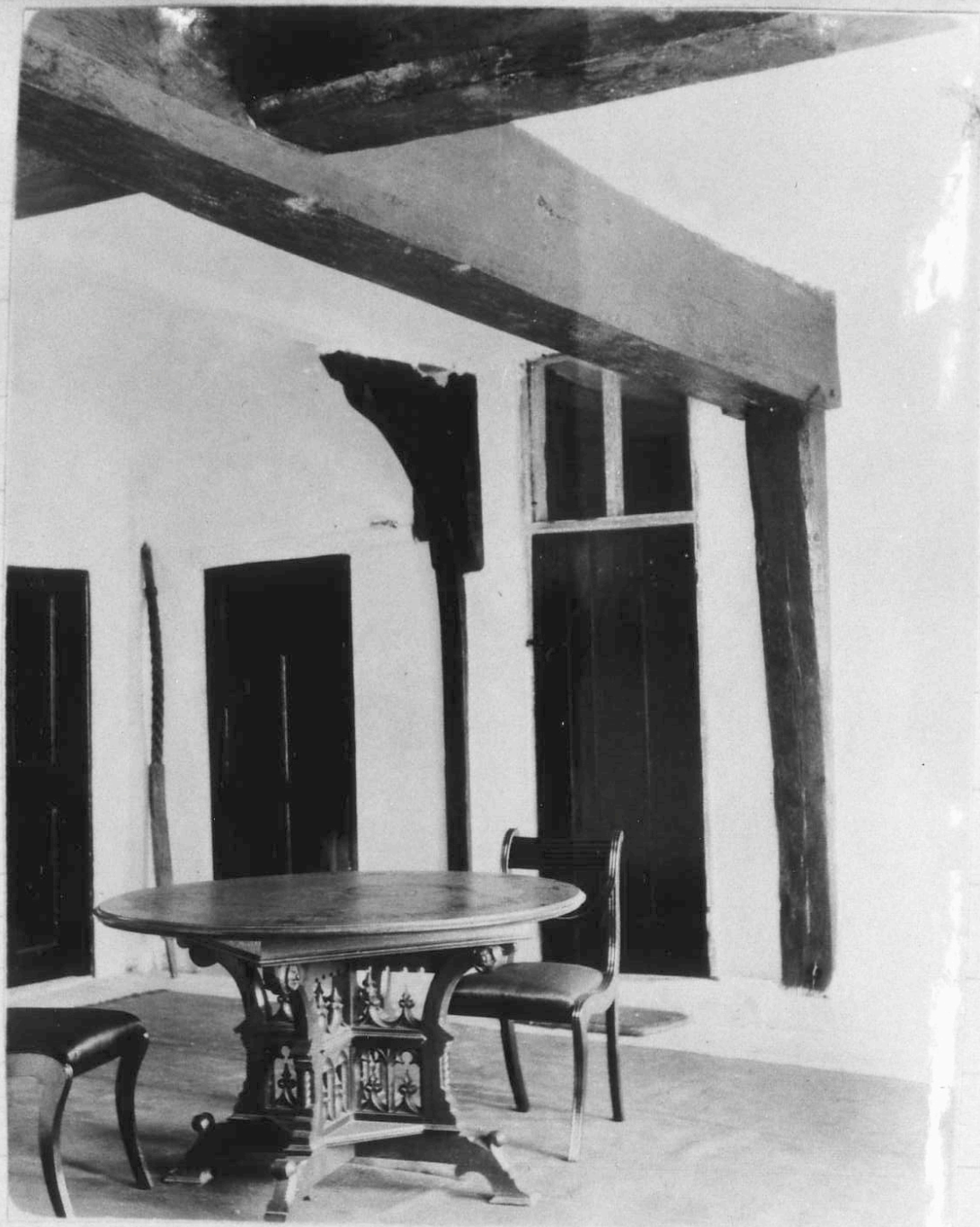
in Abbey house showing the massive oak beams
